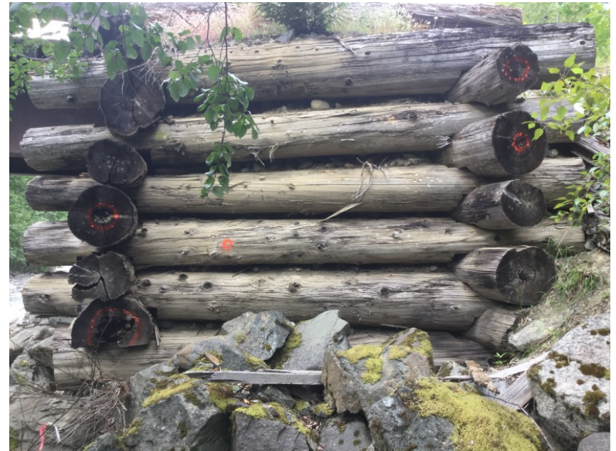
Right Abutment Upstream Wing Wall
