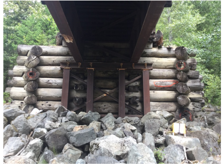
Right Bank Abutment
