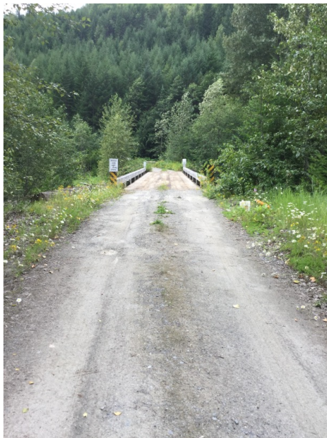
Right Approach Facing Bridge
