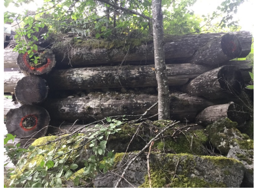
Left Abutment Downstream Wing Wall
