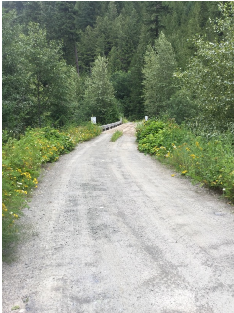
Left Approach Facing Bridge
