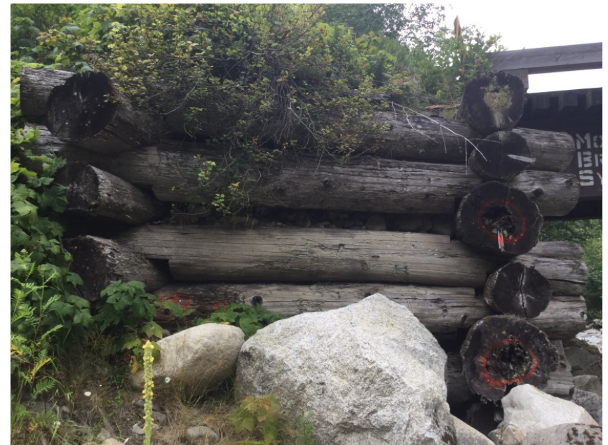
Left Abutment Upstream Wing Wall
