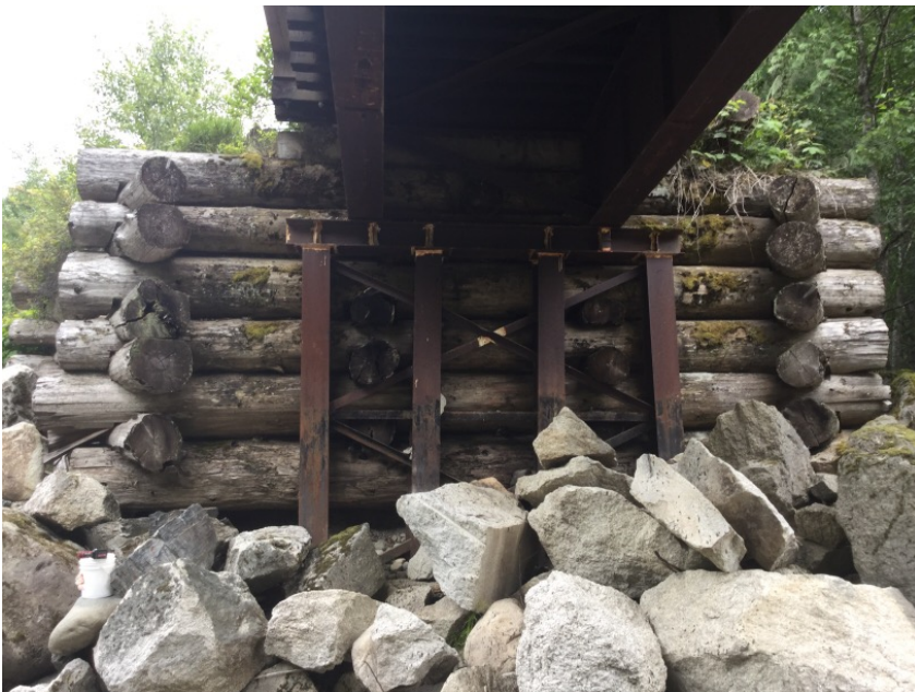
Left Bank Abutment
