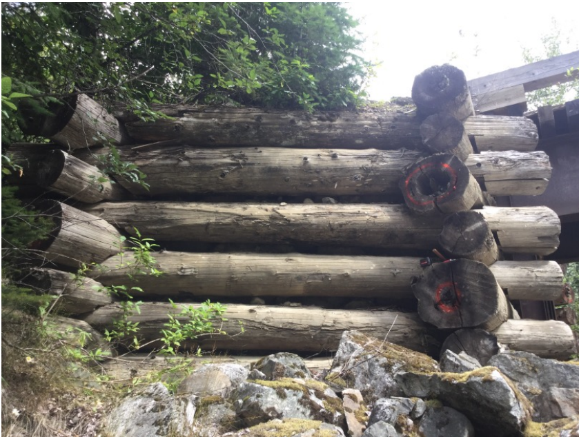
Right Abutment Downstream Wing Wall
