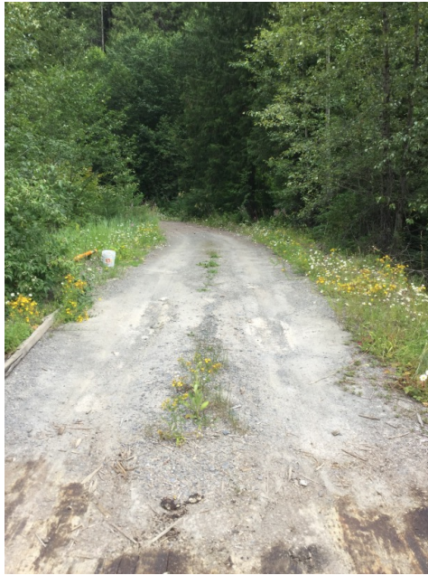
Right Approach Facing Away From Bridge
